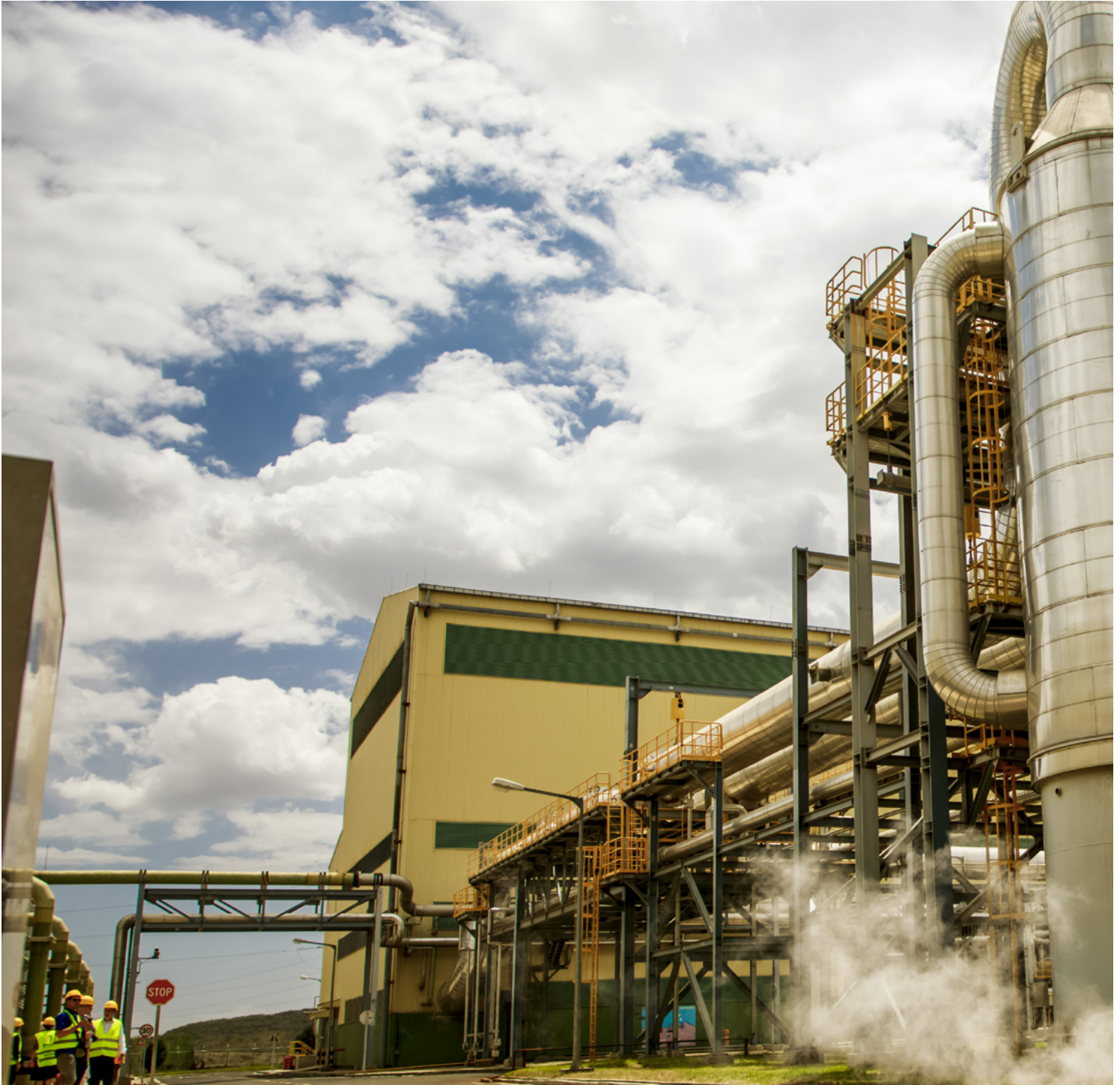
View of the geothermal power station Olkaria in KenyaUrheberrecht© Michael Gottschalk/photothek.net
