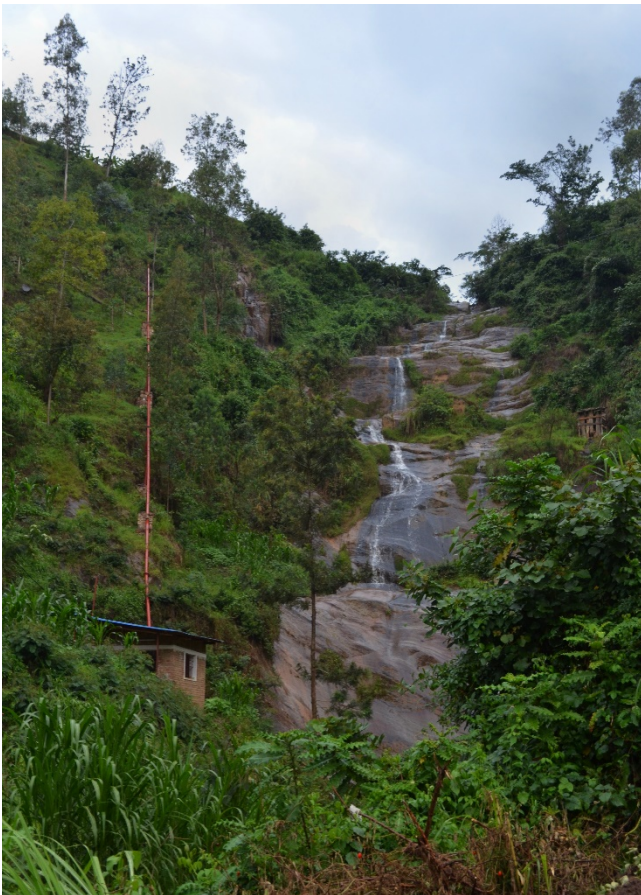
Figure 7: Power house of a 11kW hydro power mini grid.
